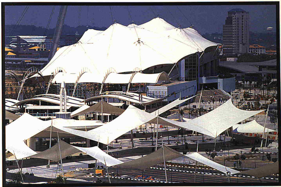
THE NATIONAL SPORTS COMPLEX IN BUKIT JALIL
